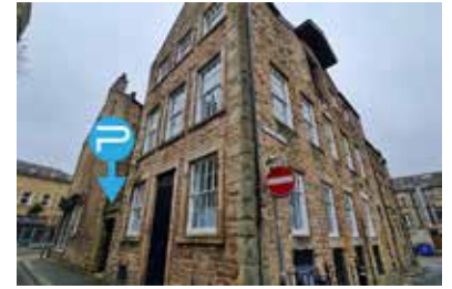
PEMFiT Entrance on Butterfield Street (Dye House Lane on the right)
