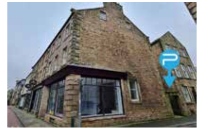
PEMFiT Entrance on Butterfield Street (Chapel Street on the left)
